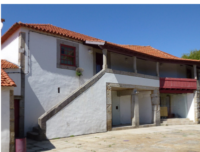
Fig. 10: Built Structure (STR), in the rural settlement of City Park.
